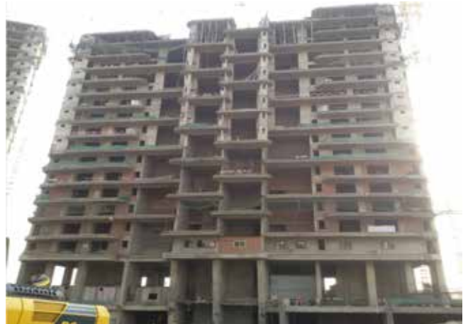
Tower 6:- 11th Floor slab completed, 6th Floor Brickwork completed
