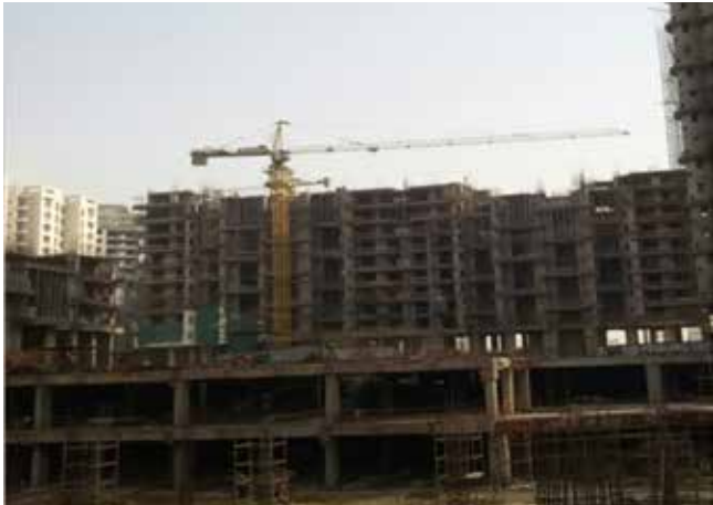
Tower 3:- 9th Floor slab completed, 6th Floor Brickwork completed
