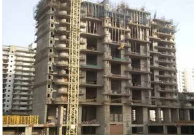
Tower 2:- 12th Floor slab completed, 2th Floor Brickwork completed
