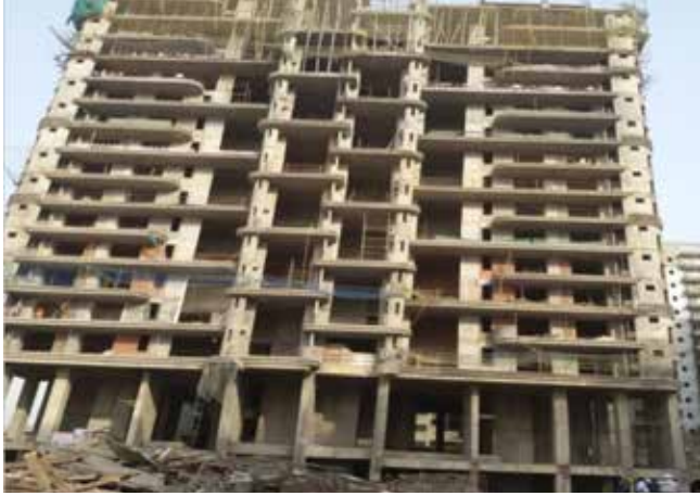
Tower 1:- 15th Floor slab completed, 9th Floor Brickwork completed
